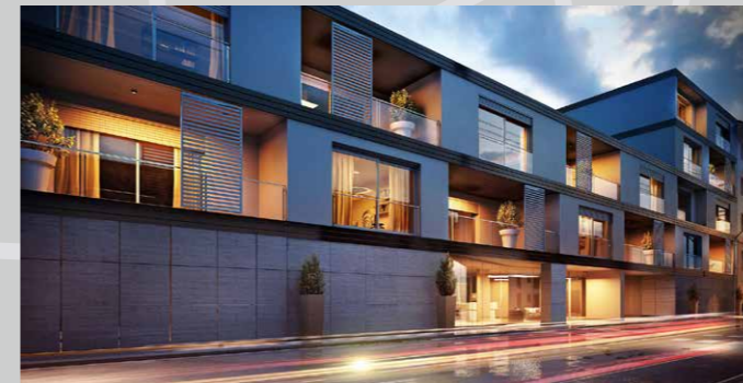
Via Isaac Newton 10, Milano 2016 Progettista / architect : LPArchitecture - Milano
