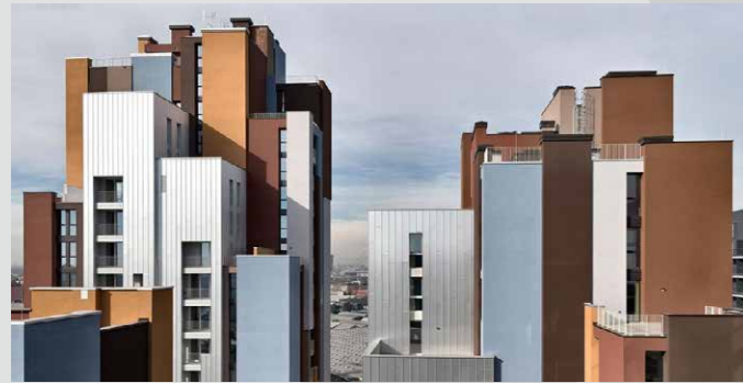
Via Gottlieb Wilhelm Daimler, Milano 2015 Progettista / architect : Mario Cucinella Architects - Bologna
