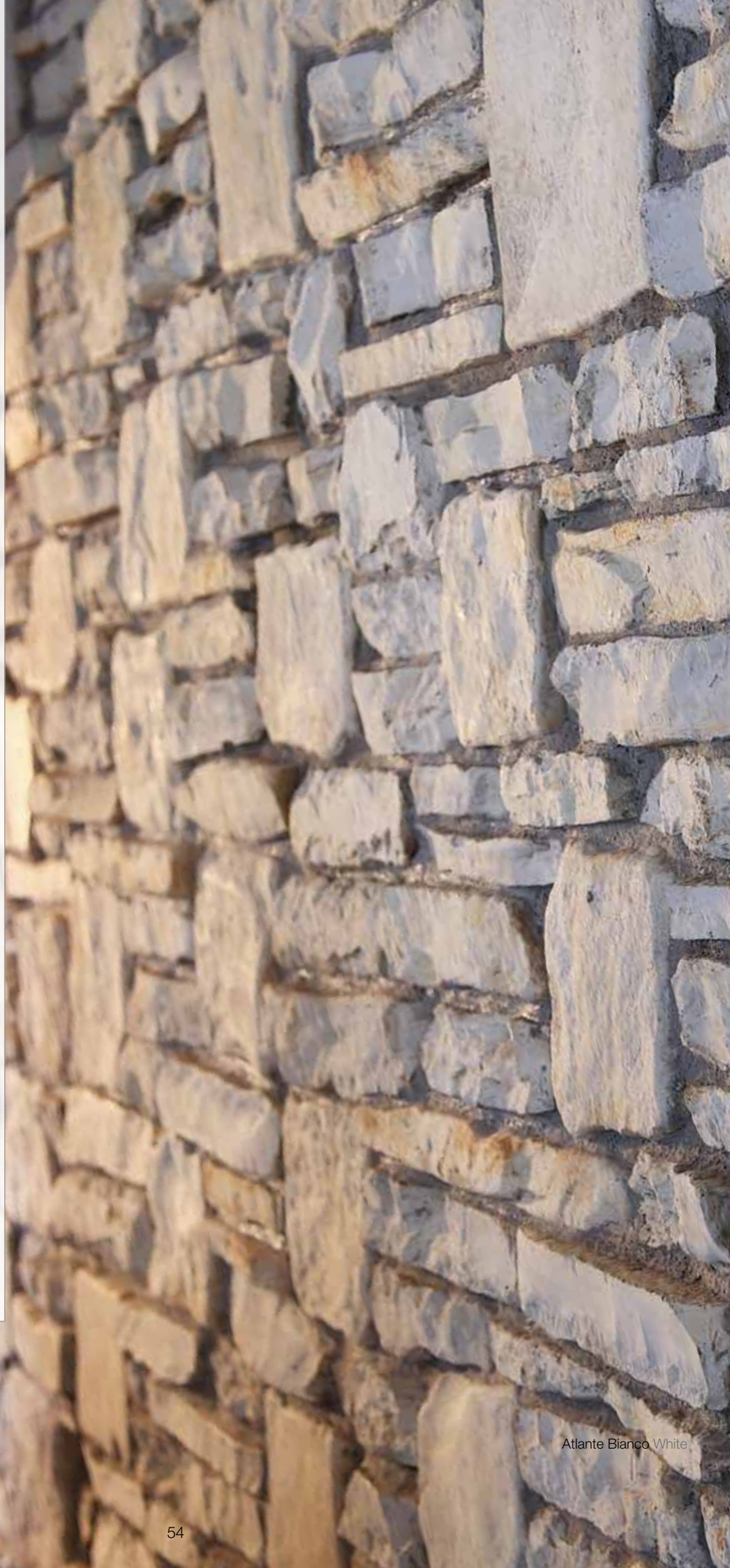
Picture above: EXAMPLE OF A MIXED STONE CLADDING (30% Yellow Alpi, 70% Yellow Ande, beige grout)
